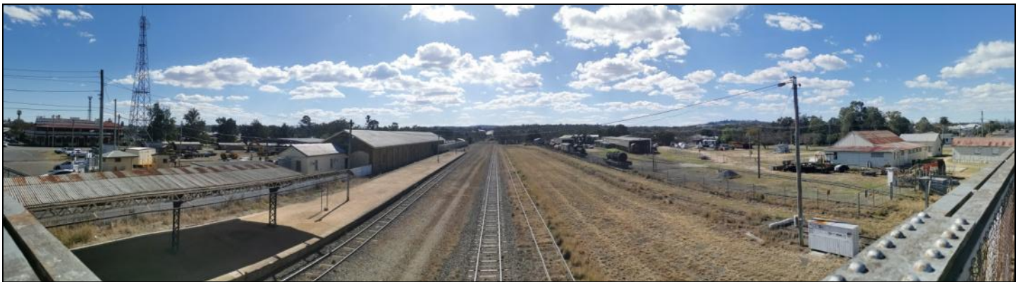
View from the bridge....left: Watco's freight hub based around the heritage sandstone goods shed. Main line North & South Right: the Railway Institute Complex and in the distance SDSR yard and maintenance facilities.
