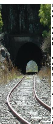
From here it is just a corner or two away from the Cherry Gully Tunnel. Construction of the tunnel started in 1878, and during construction, exceptionally hard rock was encountered. Several drilling machines failed, and hand drilling had to be resorted to.
